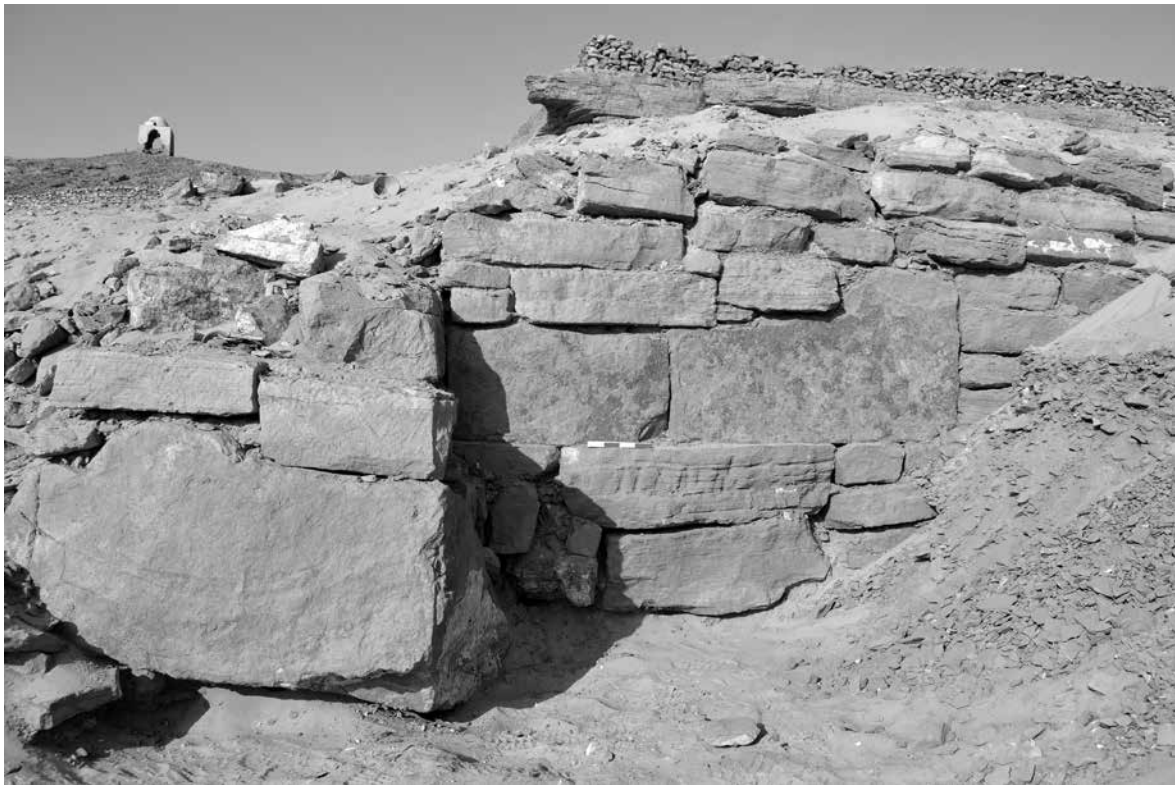
FIG. 6. Retention wall showing stepped courses, built to stabilise the area below the upper terrace of tombs.
