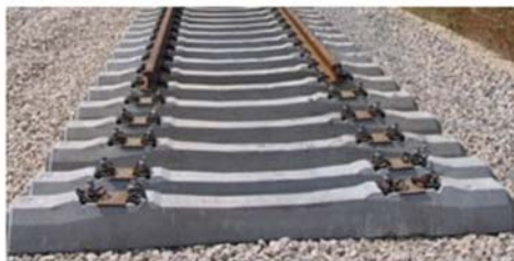
Mono Block Concrete Sleepers
