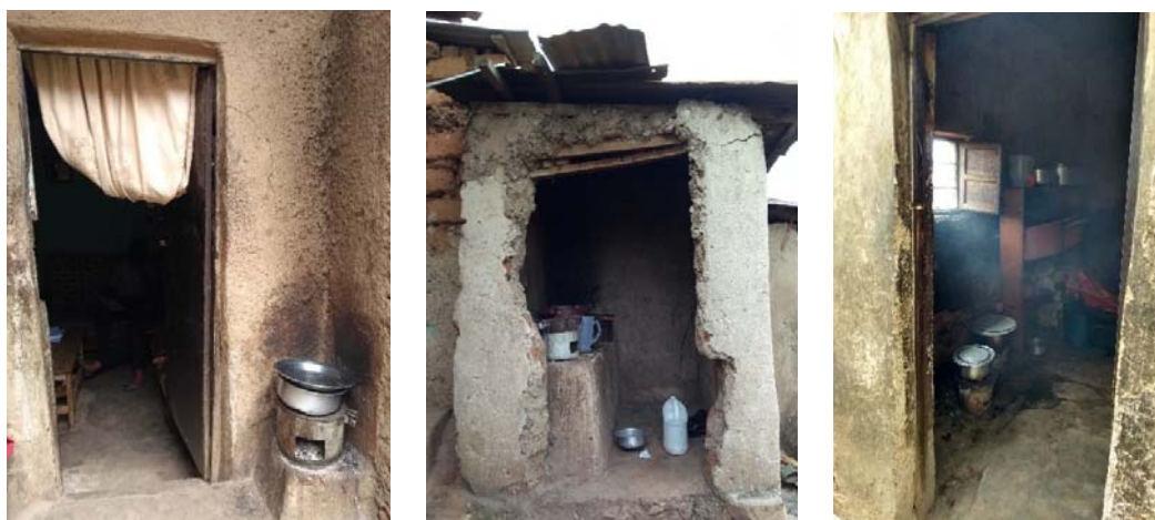
Figure 1: Typical kitchens in Muhima constructed of mud or brick on a timber frame
