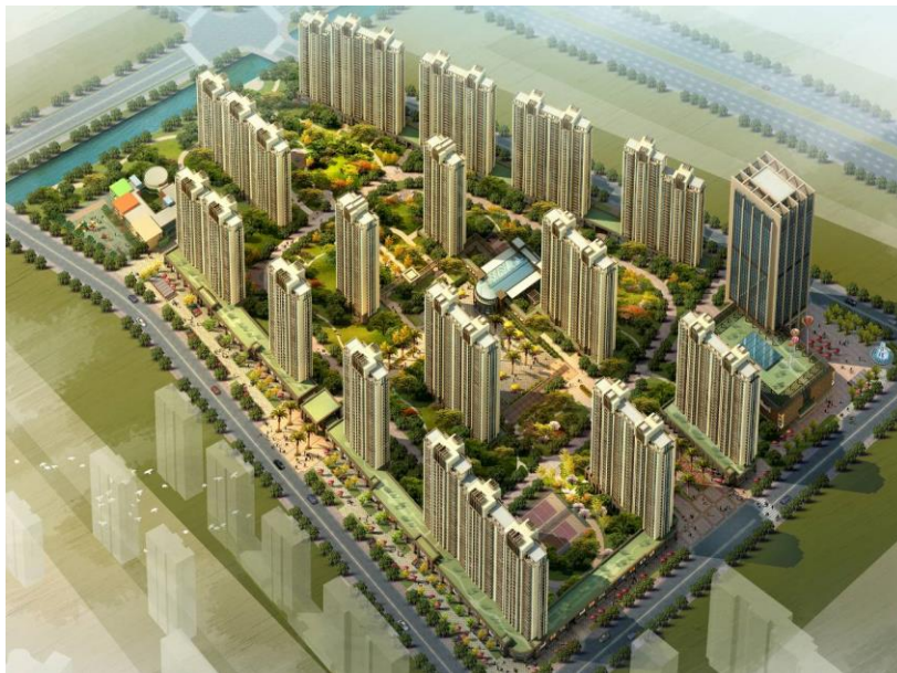
13 14 Fig. 1 A typical slab-type high-rise residential area in China, where the buildings are usually 15 assembled by 1 to 3 units, leading to plan aspect ratios ranging from 2 up to 8 or 9. 16
