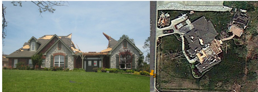
FIGURE 5 | Example of typical hip roof failure in Region 1, including an aerial photo showing the footprint of the partial failure (image source: Dr. David Prevatt, Google Earth).
