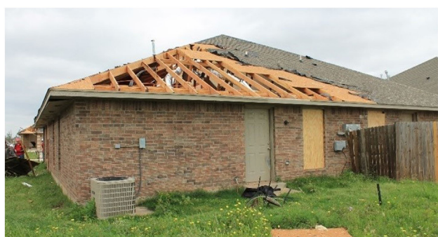
FIGURE 1 | Example of roof sheathing failure, corresponding to DOD-4 (image source: Dr. David Prevatt of University of Florida).
