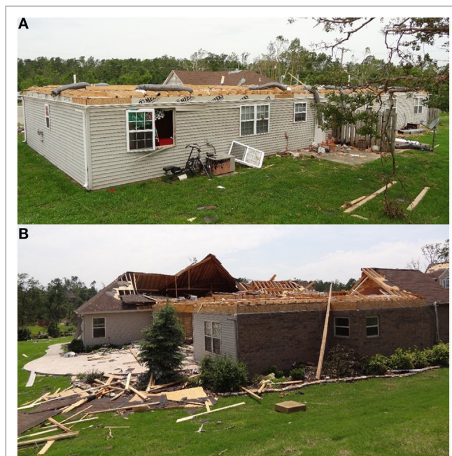
FIGURE 11 | Examples of partial stick-frame, hip roof failure with ceiling joists intact. (A) Complete removal of outer roof framing. (B) Partial removal of several faces of the roof (image source: Dr. David Prevatt).
