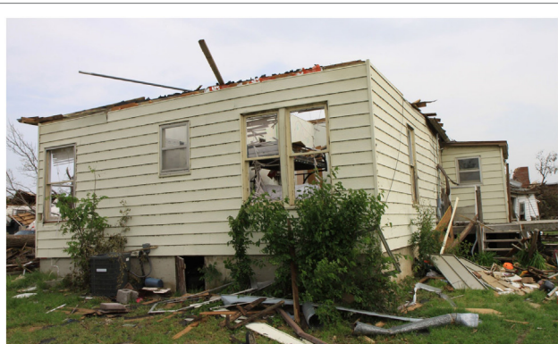
FIGURE 2 | Example of roof-to-wall-connection failure, corresponding to DOD-6 (image source: Dr. David Prevatt).
