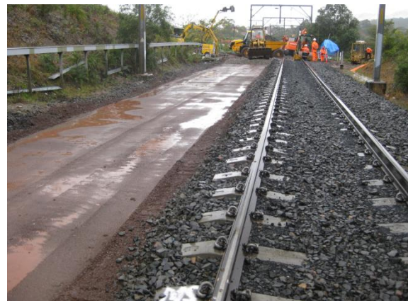
Fig. 1 Ballast and capping layer [2].
