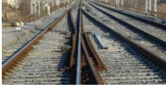
Figure 12. A typical movable crossing [30]
