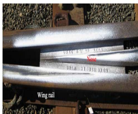
Figure 1. A standard turnout crossing nose [6]
