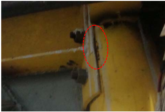
(c) Bending of extended end plate
