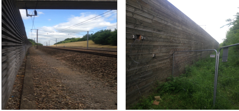
(a) Trackside view
