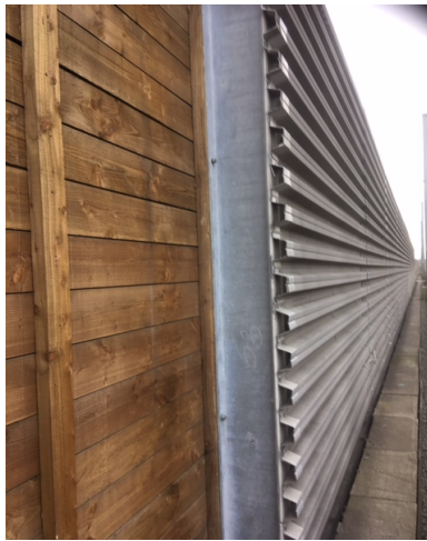
Figure 11: Difference in position from centre of track between the absorptive and reflective barriers.
