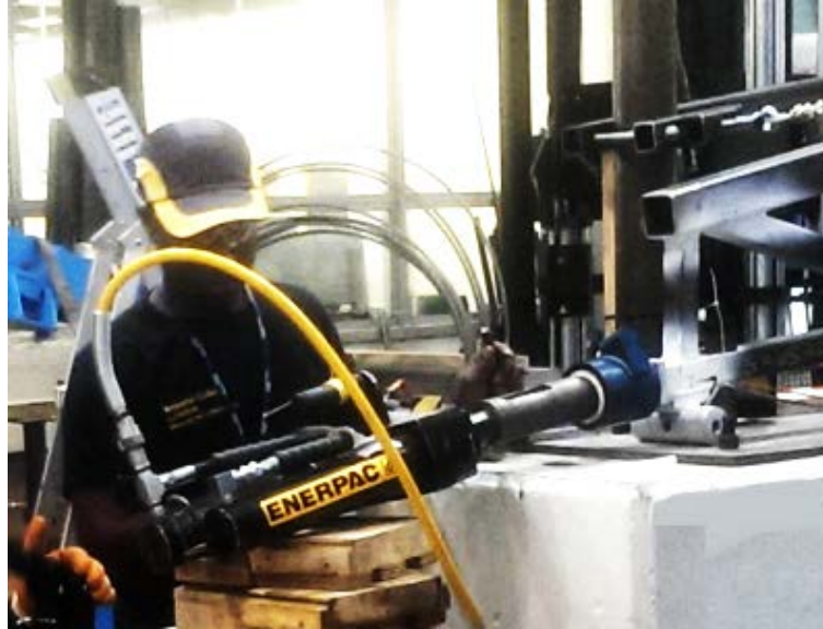
Fig. 6: Prestressing of cable
