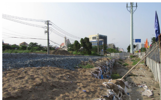
f) Increasing elevation of road redevelopment (TranNao street, district 2)
