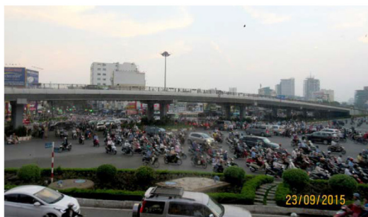
e) Overpass at Hangxanh roundabout, Binhthanh district (zone2)
