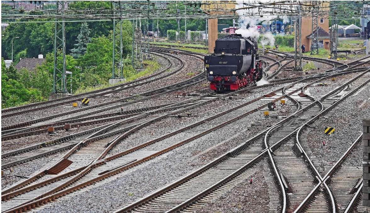
Figure 1 A widely prevalent rail junction with different kinds of turnouts
