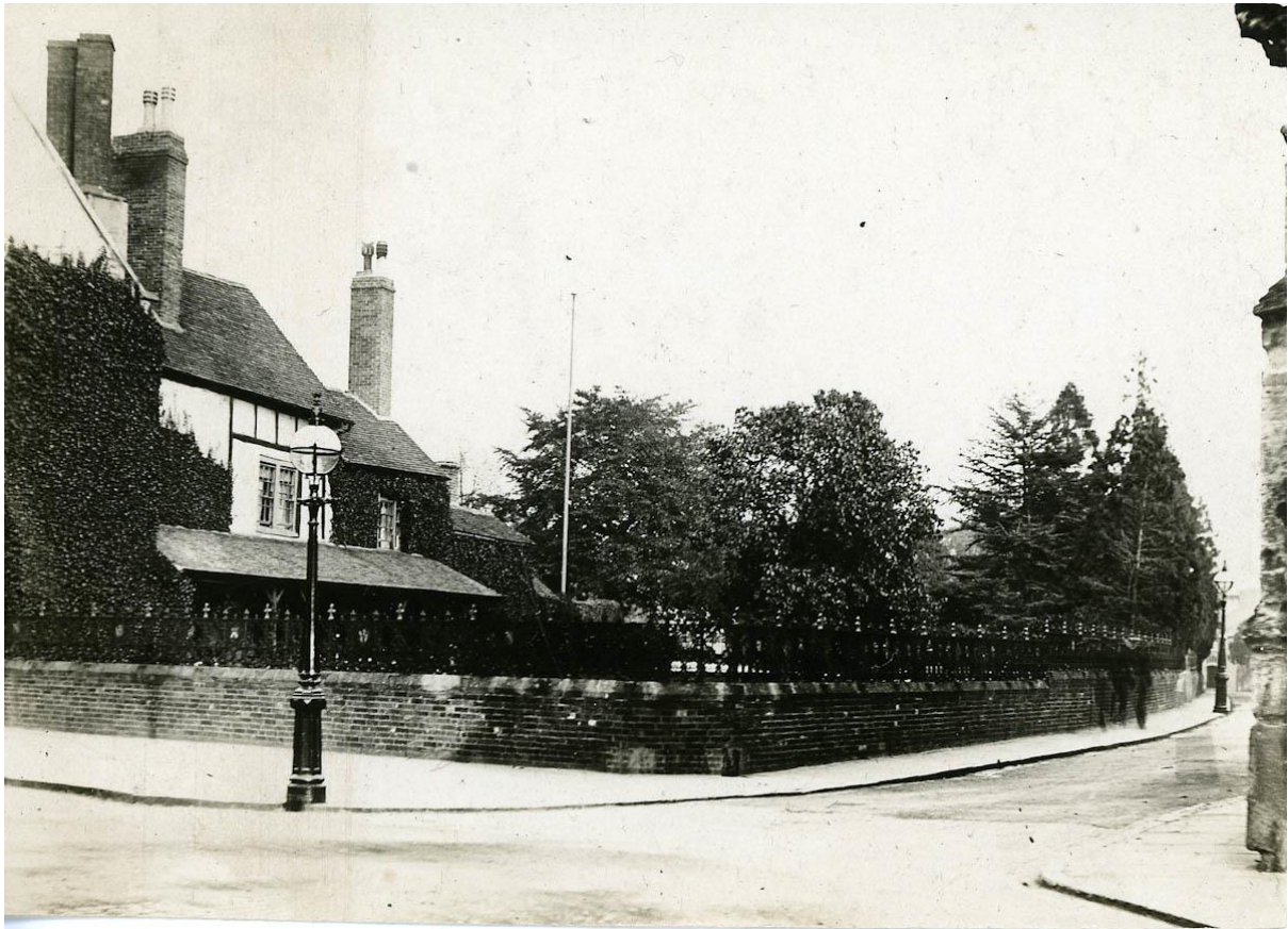
Figure 1: Chapel Street, site of New Place, c. 1900. SBT SC2/3.
