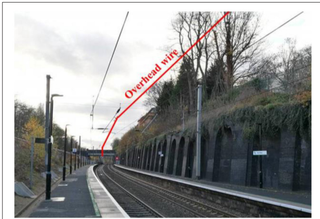
FIGURE 5 | Zig-zag path (stagger) on overhead contact wire.
