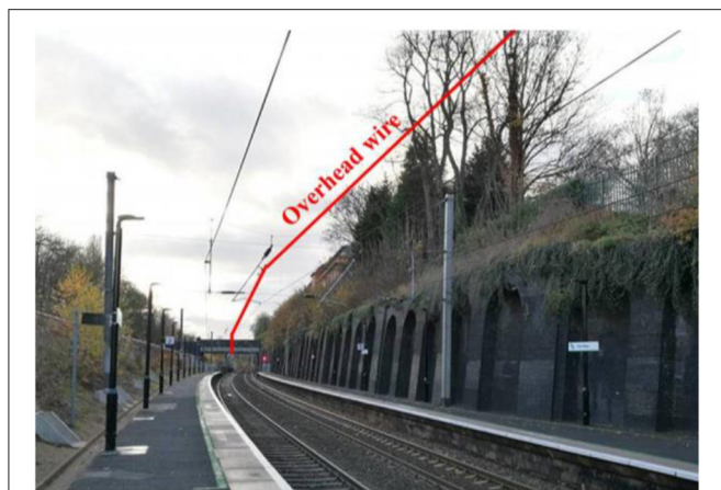
FIGURE 5 | Zig-zag path (stagger) on overhead contact wire.
