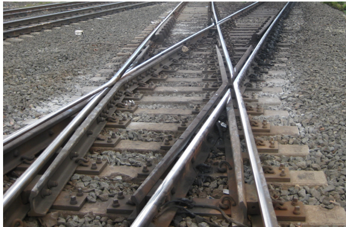
Fig. 4. Ballast pulverisation at crossing.
