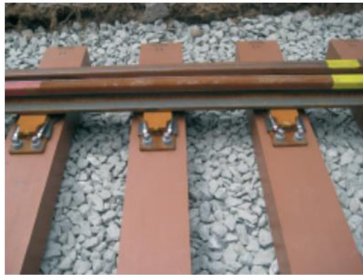
764 765 Figure 7. Composite sleepers in Zollant Bridge, Austria (SEKISUI)
