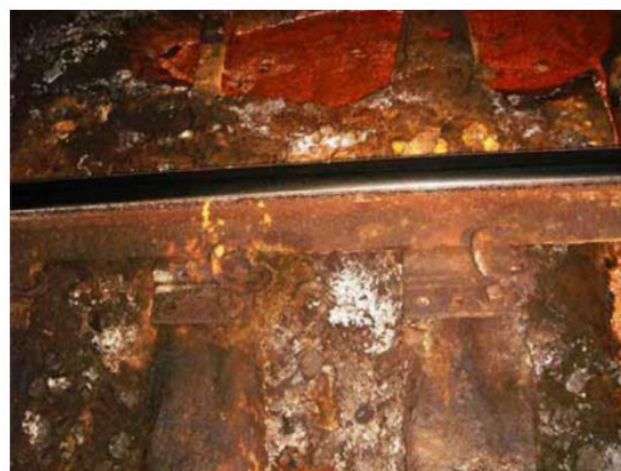
Figure 5. Corrosion in steel sleepers due salt deposits (Hernandez, Koch, and Barrera 2007)
