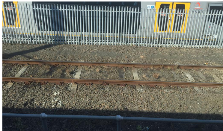
Figure 1: Deteriorated interspersed railway track (Top: mud pumping, and Bottom: ballast pulverisation and ballast dilation)
