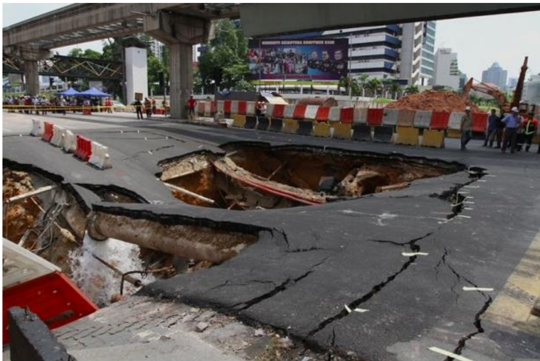
Figure 6: A 10m deep sinkhole happened in Bukit Bintang near to MRT construction (Courtesy: MRT Corp)
