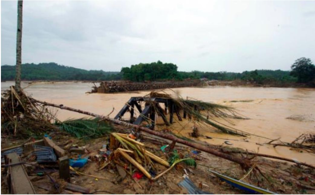
Figure 3: Malaysia East Coast Line railway bridge, which cross Nenggiri River in Kemubu, Kelantan had totally lost due to massive flood in December 2014. (Courtesy: SPAD)
