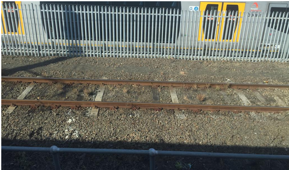
Figure 1: Deteriorated interspersed railway track (a) Top: mud pumping, and (b) Bottom: ballast pulverisation and ballast dilation
