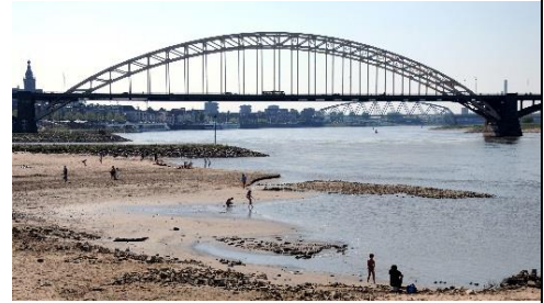
Figure B 1: 2011 drought on the River Rhine near Nijmegen (photo Ronald Puma; ronaldpuma.nl)
