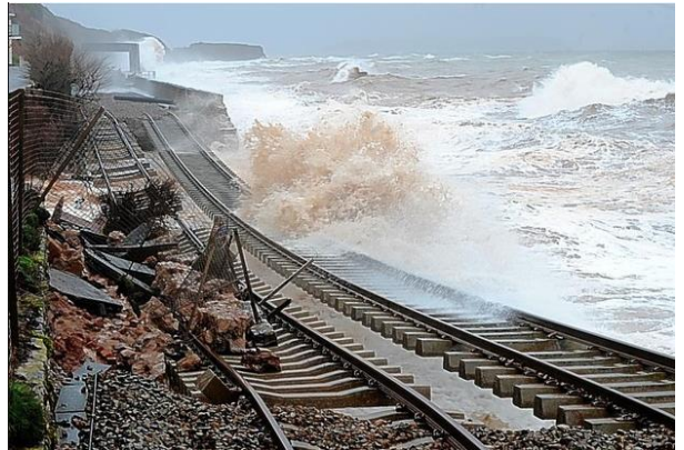
Figure 9: The main railway line to Cornwall and Devon was demolished at Dawlish by storms which hit the UK in February 2014 [15]
