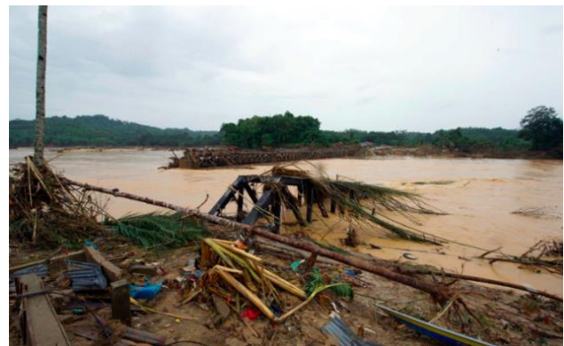
Figure 5: Malaysia East Coast Line railway bridge, which cross Nenggiri River in Kemubu, Kelantan had totally lost due to massive flood in December 2014.
