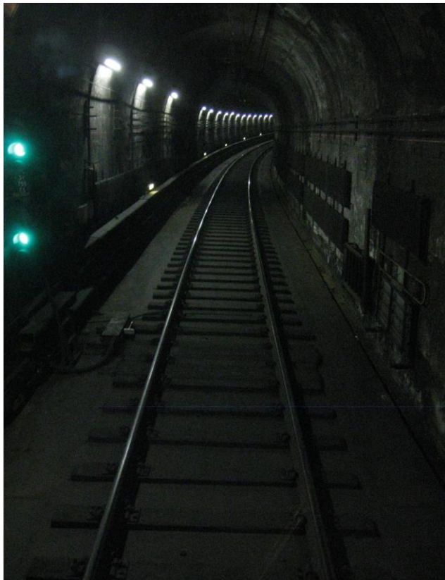
Fig. 2 A typical curved track where a high-pitch corrugation on low rail tends to occur
