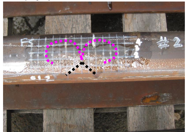
Fig. 10 Ultrasonic testing (Top: crack depths at each grid; Bottom: top view rail surface)
