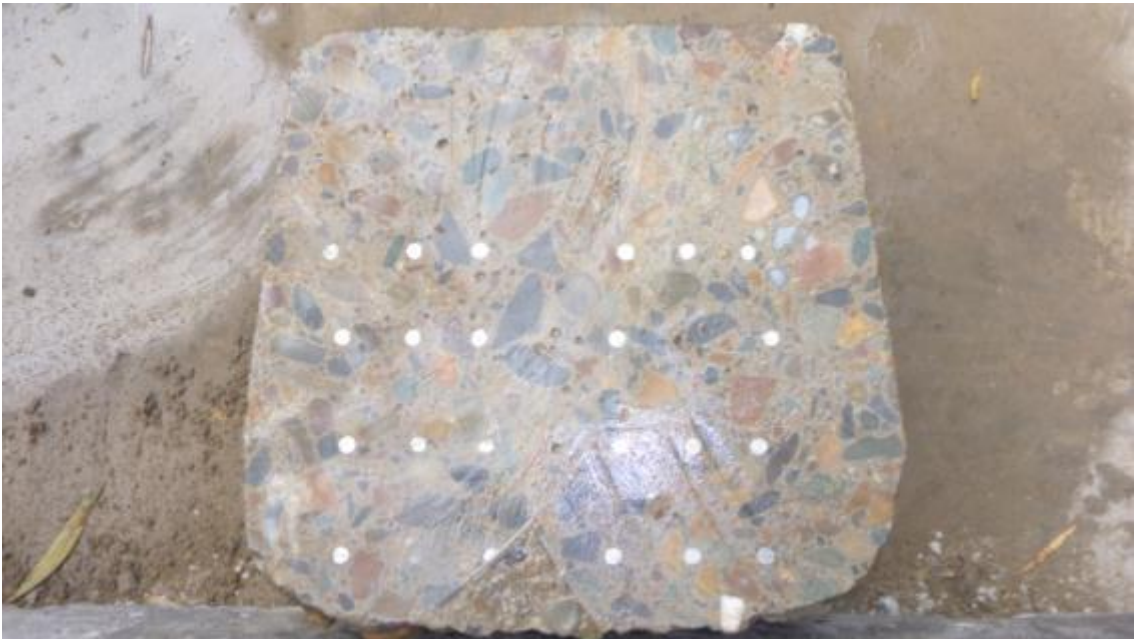
Figure 4. Freshly cut sleeper end ready for coring (SRA1)
