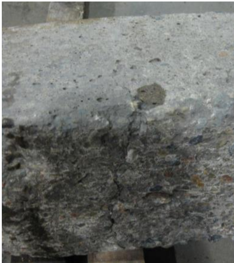
f) a wide crack underneath the rail seat of sleeper UOW6
