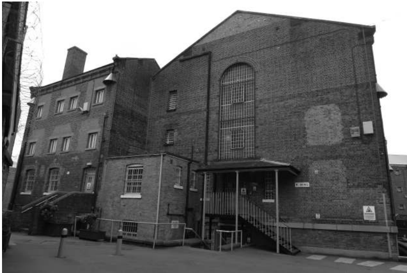
Fig. 3 Exterior view of HMP Wandsworth, London (1851)
