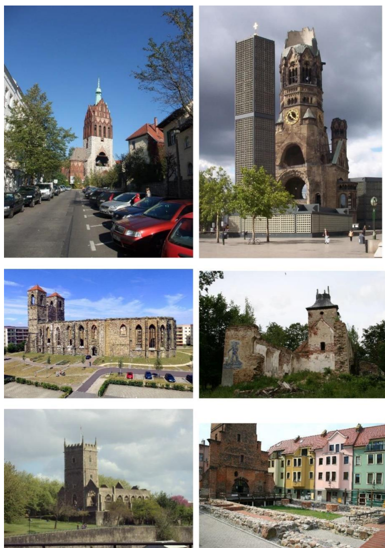
Figure 4. War-damaged churches. Top left: Bethanienkirche, Mirbachplatz, Berlin: a prominent location (photograph by Sebastian Wallroth, CC-BY-SA-4.0). Top right: Kaiser-Wilhelm-Gedächtniskirche, Berlin-Charlottenburg, a national memorial function (photograph by Null8fuffzehn, German Wikipedia). Centre left: St Nikolai, Zerst, ruin in the centre of a rebuilt residential area (photograph by Bodow, CC-BY-SA-4.0). Centre right: rural ruin of Borchersdorf-Selenopolje, Kaliningrad Oblast (photograph by Kno-Biesdorf, CC-BY-SA-4.0). Bottom left: St Peter, Bristol, ruin in a new urban city-centre park (photograph by Rept0n1x, CC-BY-SA-3.0). Bottom right, ruins of St Catharine's church, Bytów, surrounded by historicist reconstruction (photograph by Danapass CC-BY-SA-3.0-PL).
