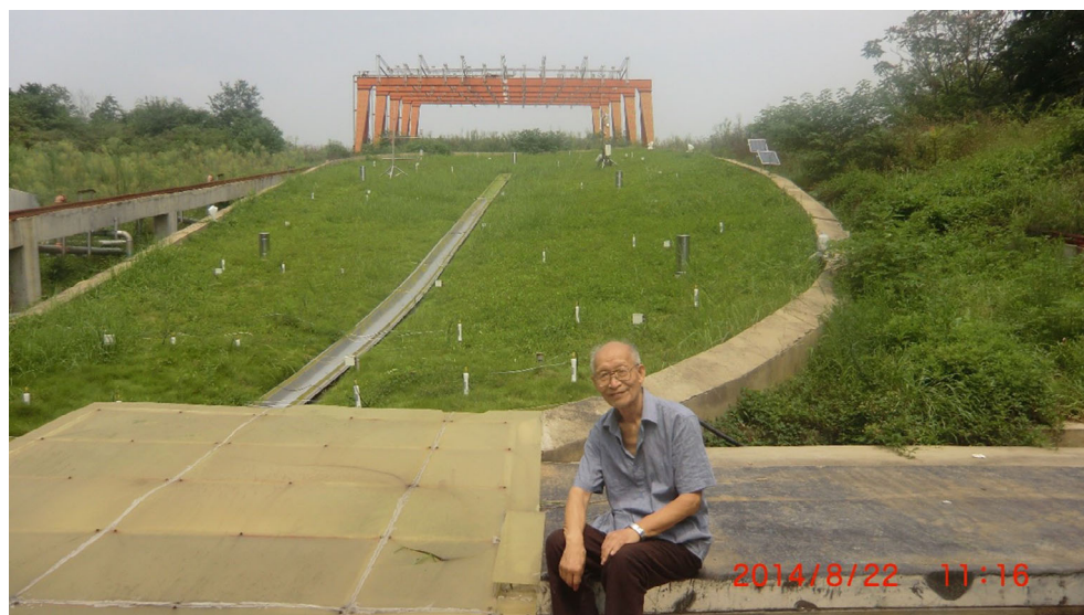
FIGURE 1 Prof. Gu at Hydrohill. This 490 m 2 catchment took 100 workers 5 years to construct, according to the many early conversations, I had with Gu in Nanjing in the 1990s. Source: Aimin Liao.
