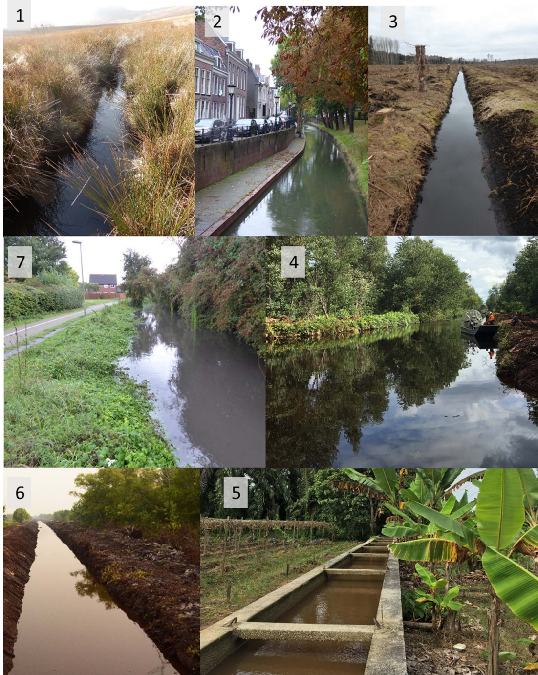
Figure 1. Photographs of ditches differing in design and function. Clockwise from top left: (1) ditch in a UK upland blanket bog; (2) an urban canal in the Netherlands; (3) a ditch in a felled peatland forest in Sweden; (4) a water management channel in an Indonesian Acacia plantation; (5) a rice paddy irrigation channel in Malaysia; (6) a freshly dug ditch on ex-Mega Rice Project land in Central Kalimantan; (7) a UK urban ditch under flood conditions.
