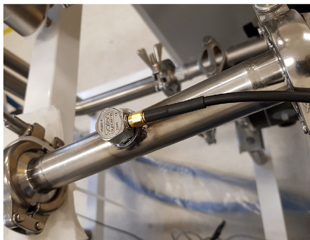
FIGURE 2 Top view on the pipe segment with acoustic emission (AE) sensor (sensor flange removed).
