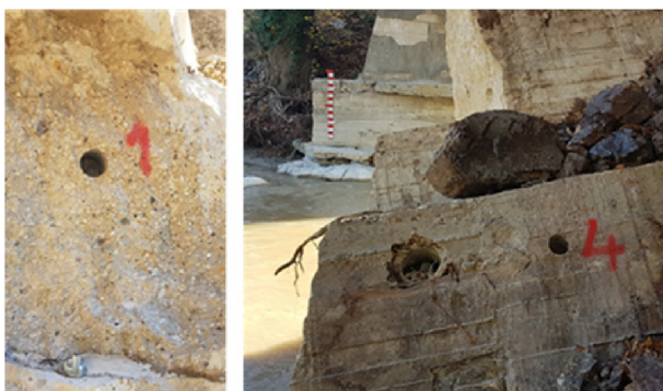
Fig. 6. Photos of core extraction locations.
