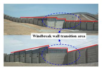
Figure 1. Windbreak transitions in the railway.
