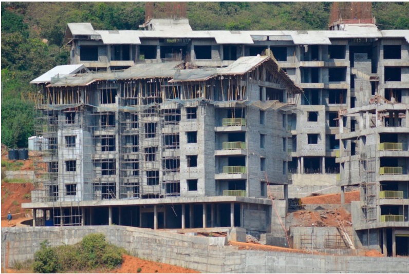
Figure 1. Photograph showing a building under construction, Source: photograph by author.
