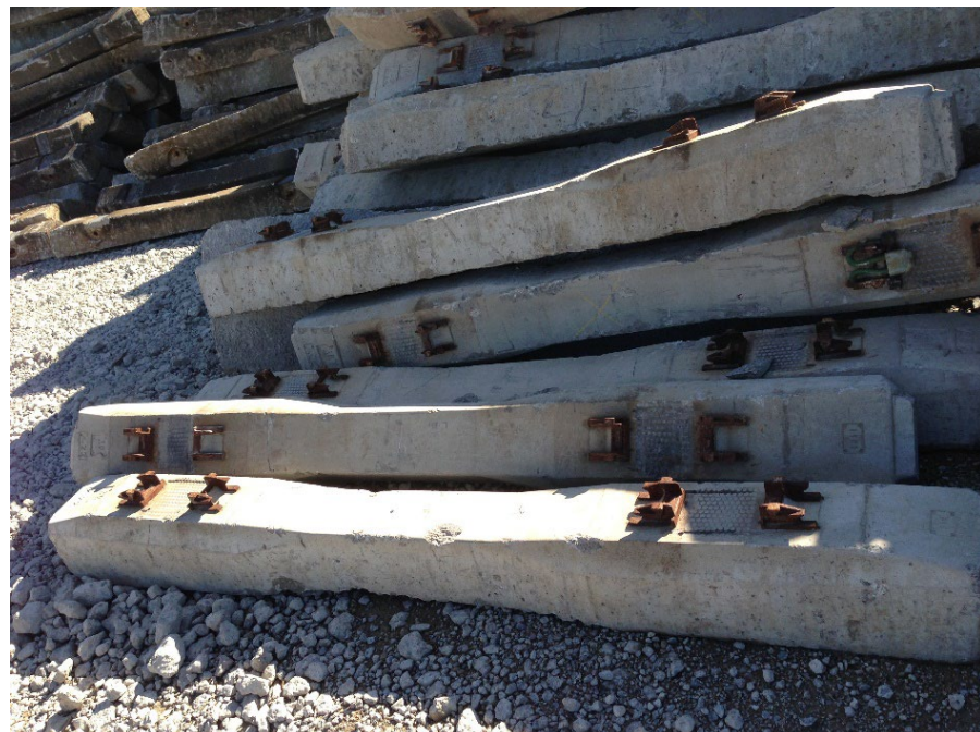
Figure 1. End-of-life railway prestressed concrete sleepers. Concrete is relatively intact in many sleepers after 50 years, raising a concern for better design optimisation. (Courtesy: Abetong AB)
