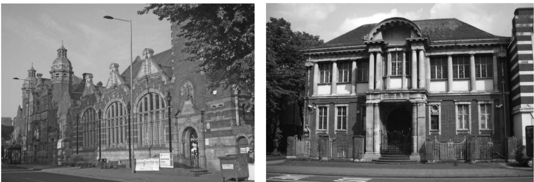
Figure 2. Moseley road baths and library (left): an architectural ensemble of Edwardian grandeur (authors’ photograph, 2018). Balsall Heath college of art (right): part of the public building ensemble (photograph by Oosoom at English Wikipedia).
