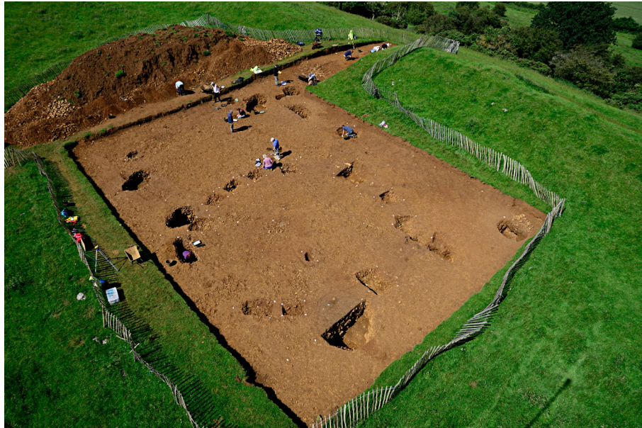
Fig. 5. View of trench 6 under excavation with the roundhouse and associated pits, many of which were lined with the sampled clays.
